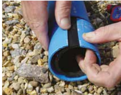
Pull the peeled layer.
