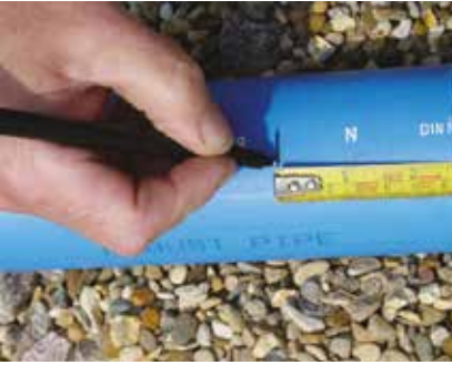
Measure and mark the pipe.
