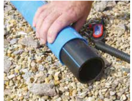
The inner layer is ready for smoothing and soldering(welding).
