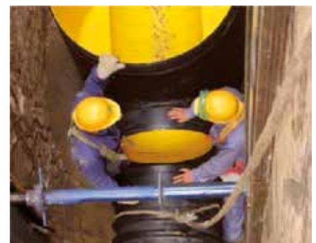
Electric fusion welding of a manhole and a pipe
