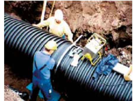
Process of electric fusion welding
