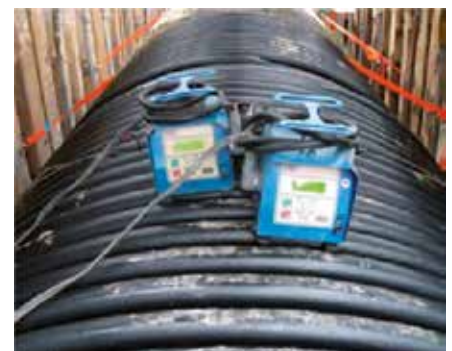
Electric fusion welding of a large-size pipe in a narrow trench
